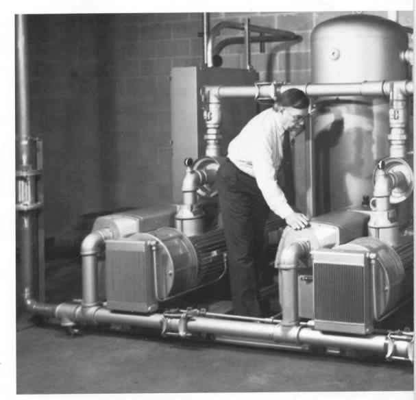
Walter Enderley, collating manager of the Newsday newspaper, checks the operation of the paper's centralized vacuum system. The four pumps, including a backup, operate in a rotating cycle to ensure reliability.
